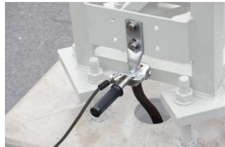
Earth connection with universal clamp
